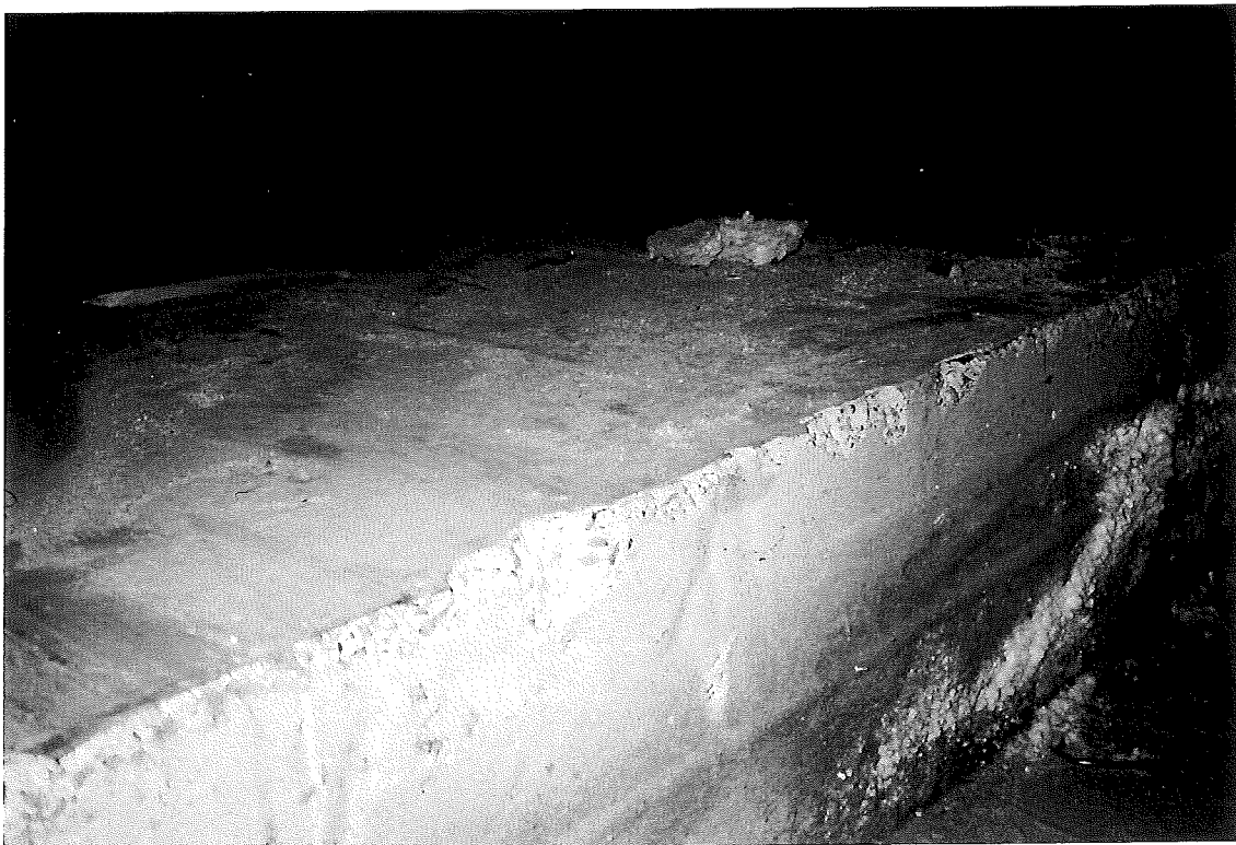
PHOTO 4: Asbestos-containing 9" Floor Tile and Ceiling Material debris Crawl Space below Dining Area
