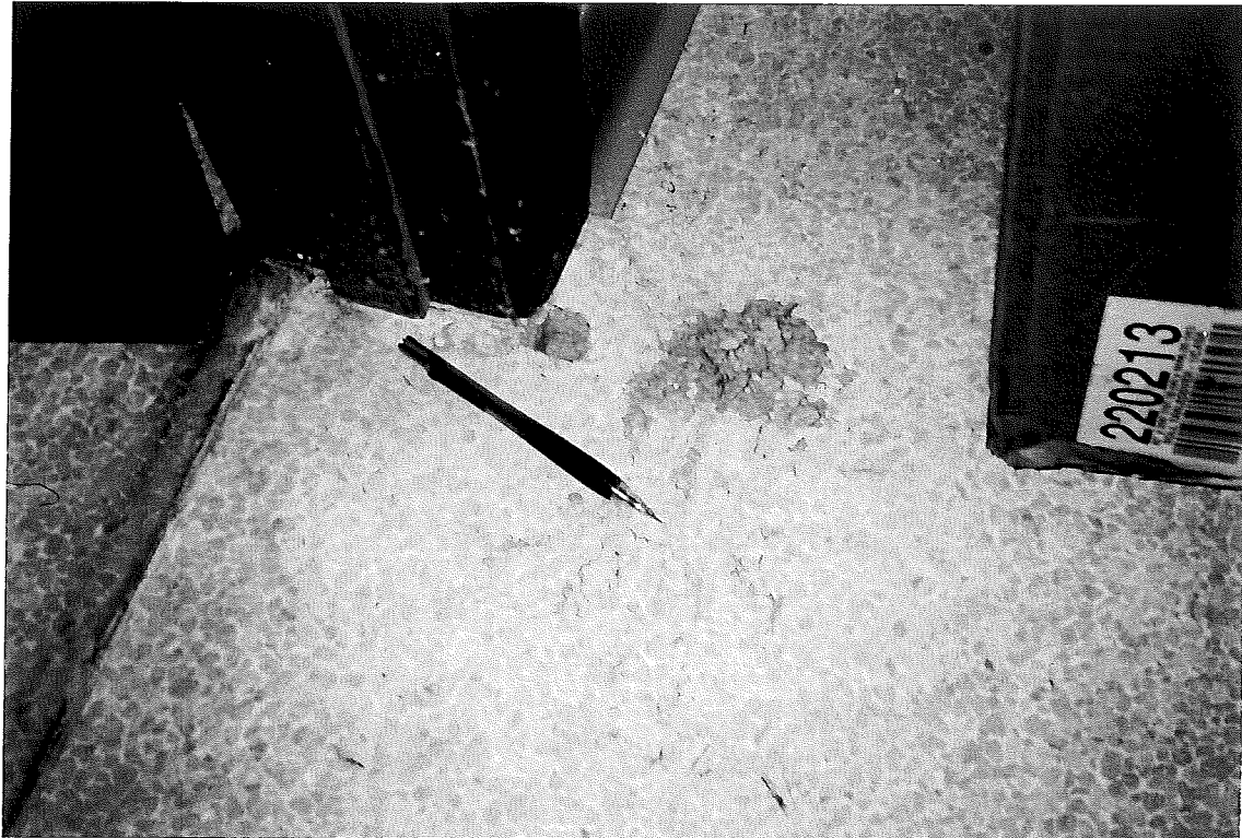
PHOTO 2: Layered Floor System in Dining Area Top Sheet Vinyl layer (1) and Particleboard conceal Asbestos-Containing Sheet Vinyl (2)
