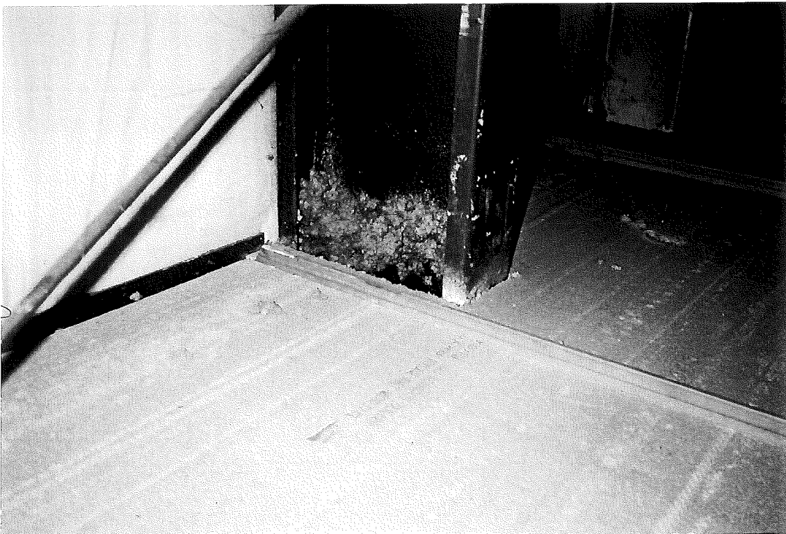
PHOTO 6: Remnant Asbestos-containing Sprayed-on Ceiling Material Above Drop Ceiling- South Perimeter Column
