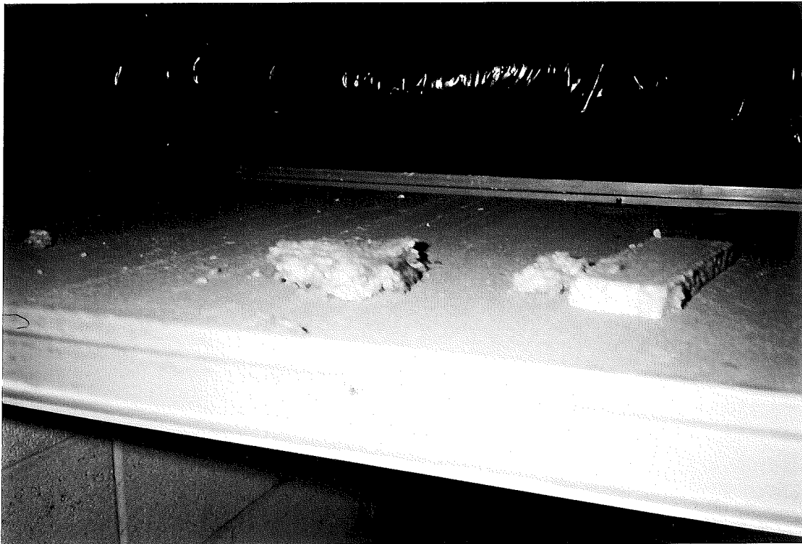
PHOTO 5: Asbestos-containing Sprayed-on Ceiling Material Debris Above Drop Ceiling in Kitchen Area
