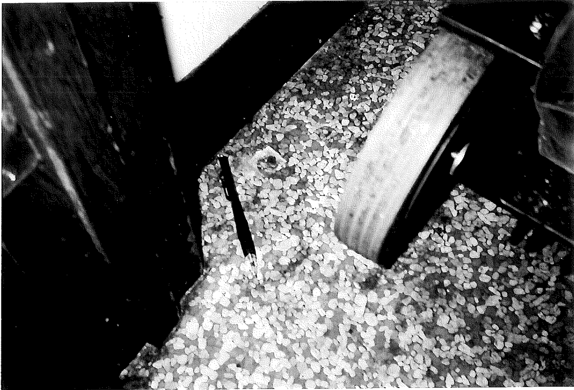
PHOTO 3: Asbestos-containing Vinyl Sheet Flooring (3) Janitorial Closet
