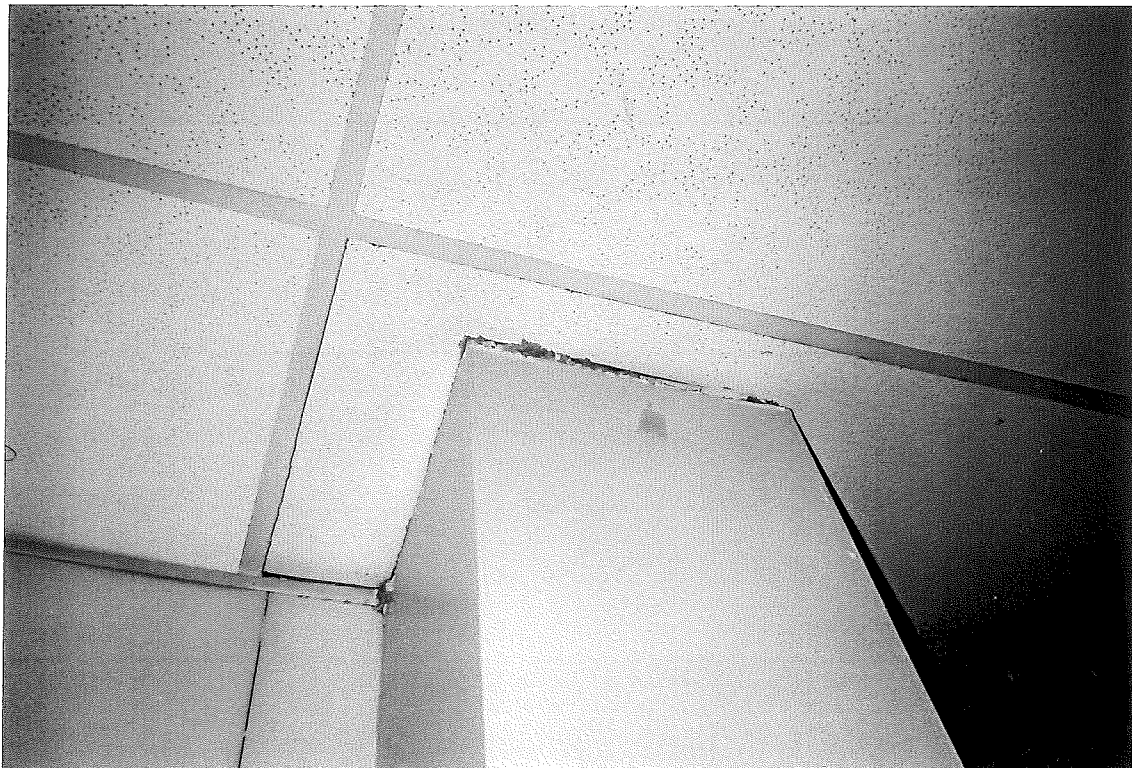
PHOTO 8: Remnant Asbestos-containing Sprayed-on Ceiling Material Perimeter Column Soffit
