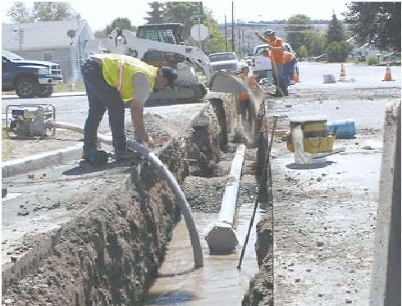
Crews removed the last wooden water line during FY 24 Q1 – Photo: Jason Chaney/The Central Oregonian
