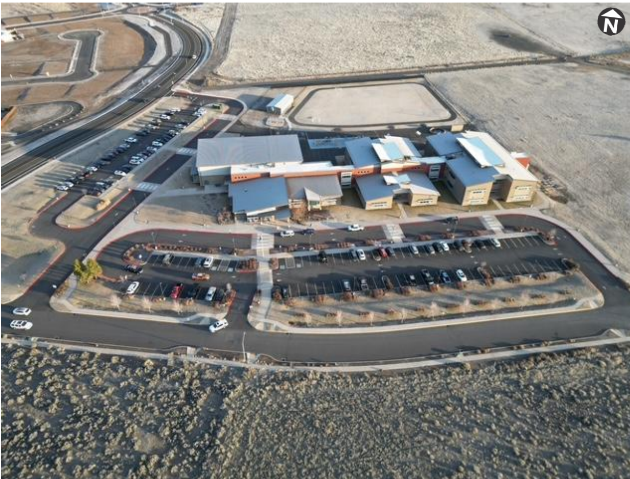
Figure 15. Barnes Butte Elementary School Layout. Photo date: February 12, 2026.
