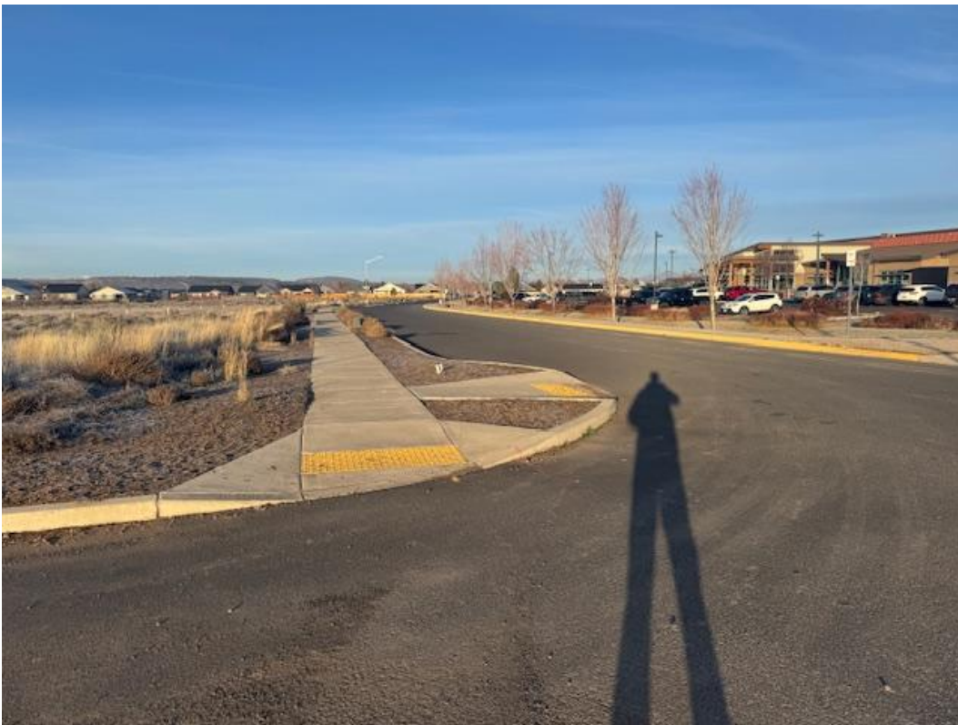
Figure 12. View from the eastern street connection facing west. Photo date: February 2026.
