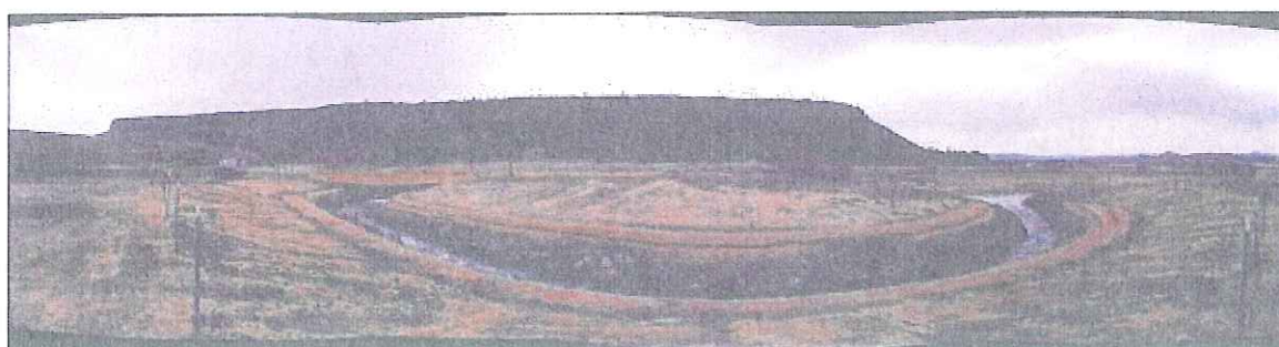
Fish bypass channel around diversion dam
