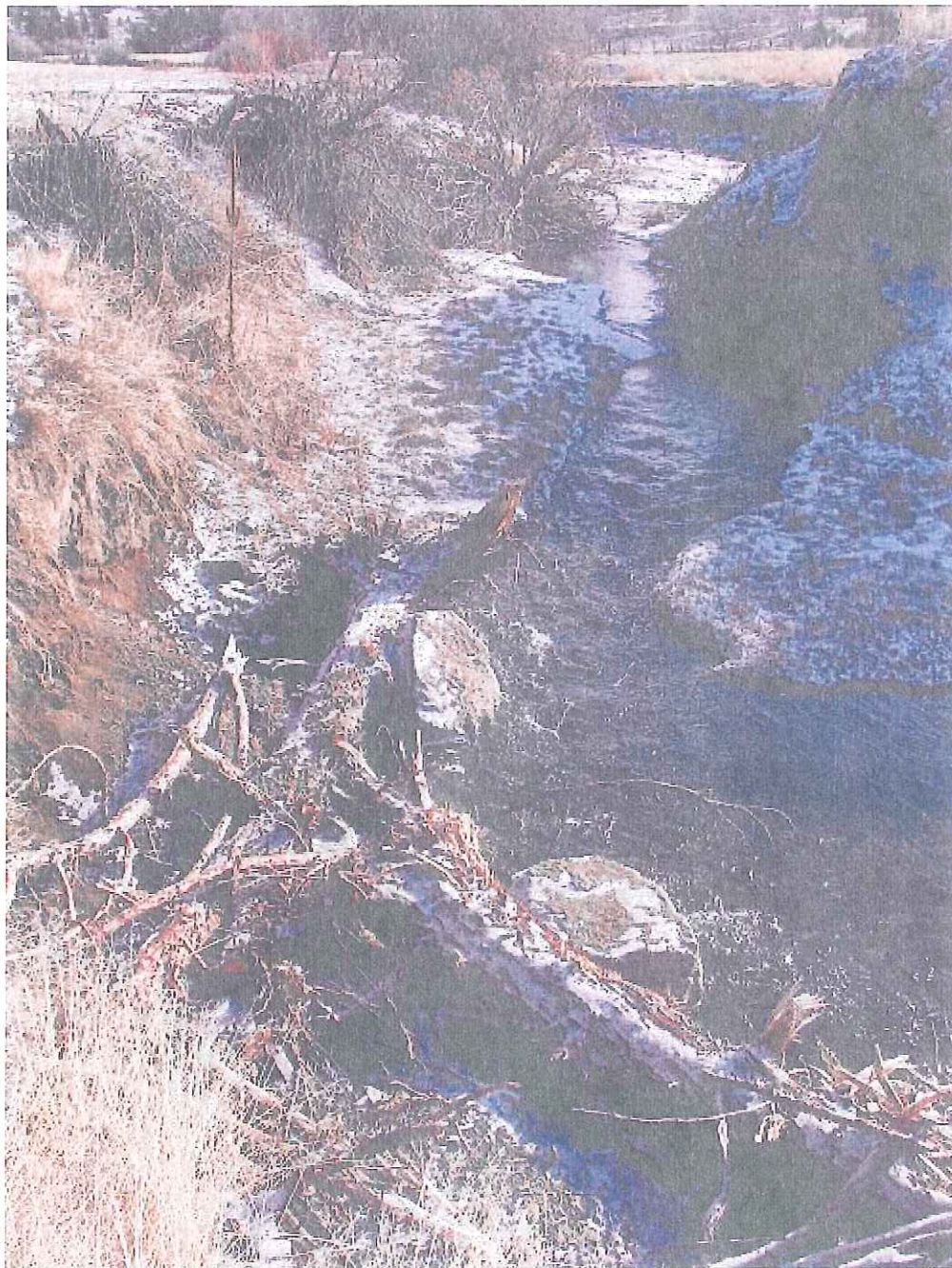
Bank stability structures to reduce erosion
